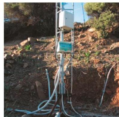
The foundation is made by pouring concrete blocks with a volume of 1 m<sup>3</sup> each for the stays and the mast foot. The concrete foundations must be laid in the earth so as to be frost-free, depending on the height of the mast, at a defined distance from the mast and flush with ground level. Allow the concrete to set properly before the mast is erected.
